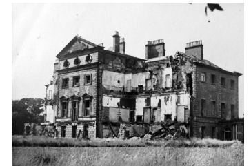
Lathom Hall during demolition in 1925
